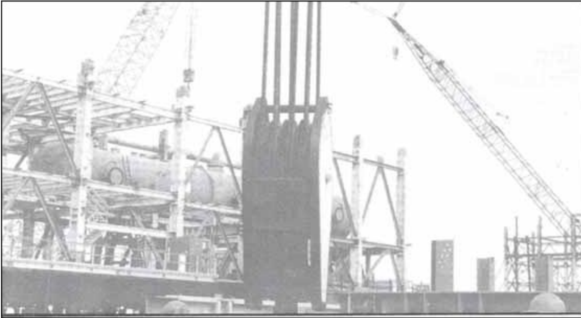
Typical Construction Site Load Block Lowered for Inspection
