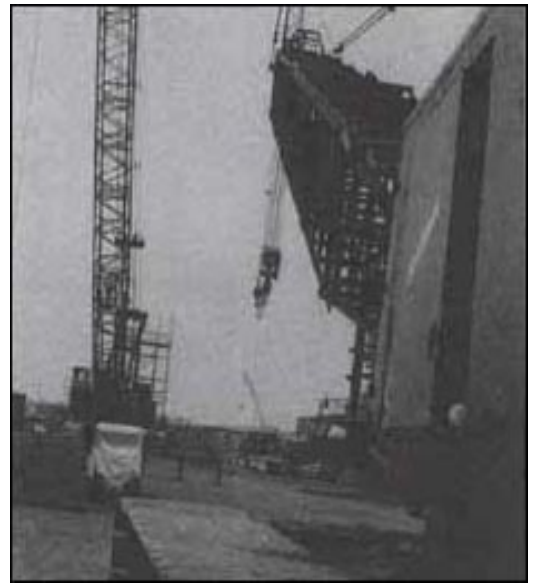
Crawler Crane Prepared for Inspection
